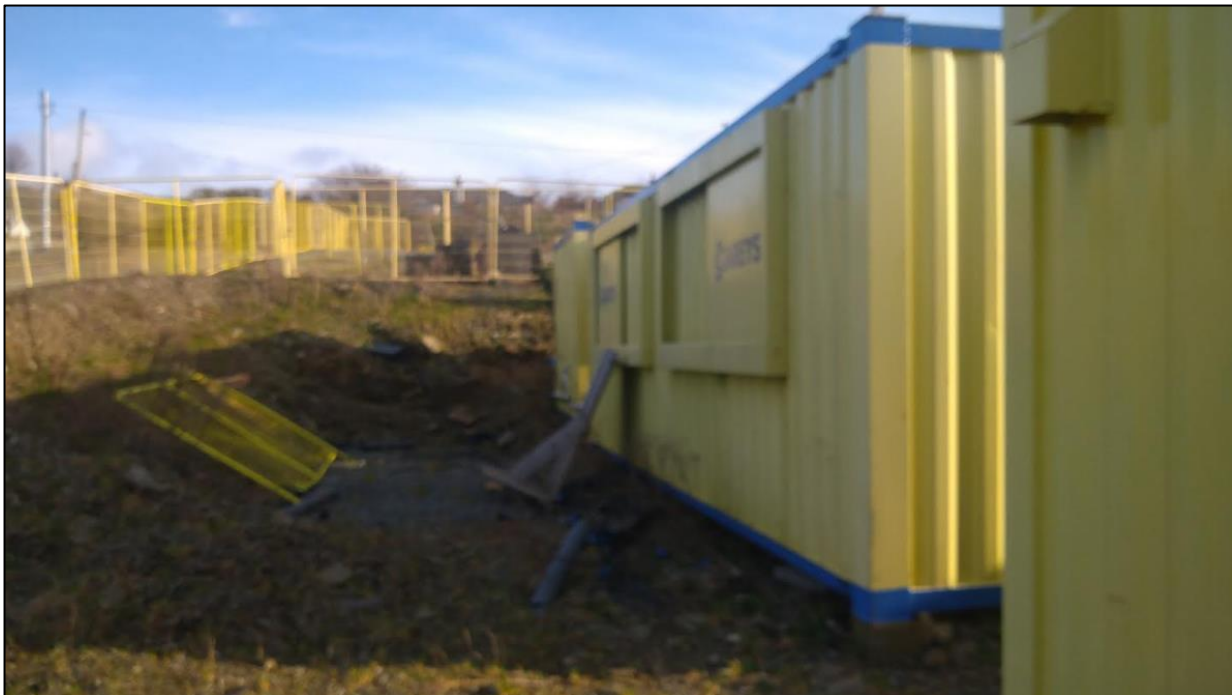
Plate 4: Note depth of ground reduction for compound.
